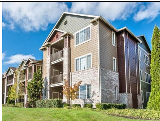
FIGURE 702-6. EXAMPLE OF DESIGN ELEMENTS FOR ARTICULATION
