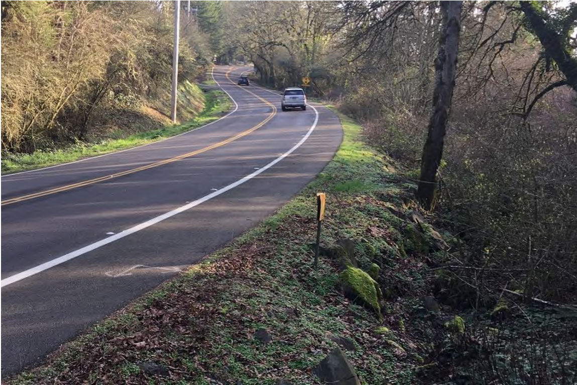
Figure 14. View Facing South from the Proposed Access on Doaks Ferry Road.
