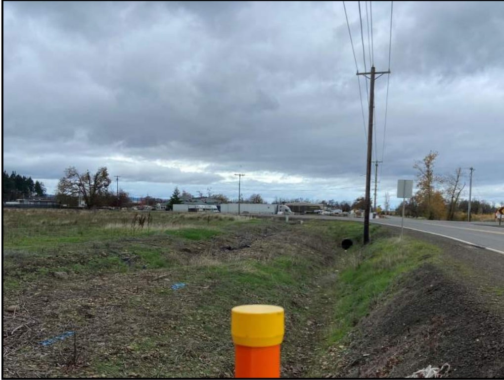
Figure 9: Site Access #2 (South Driveway) Looking North
