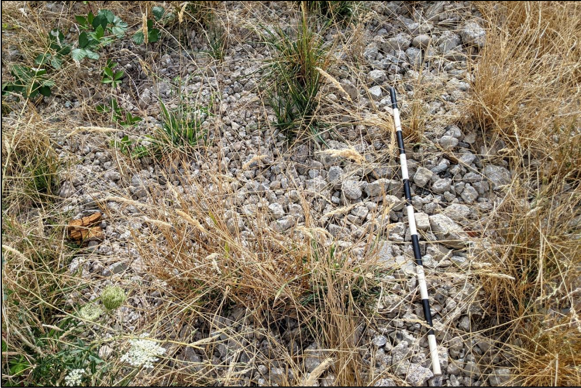
Figure 20. Concrete rubble surface typical across the project area.
