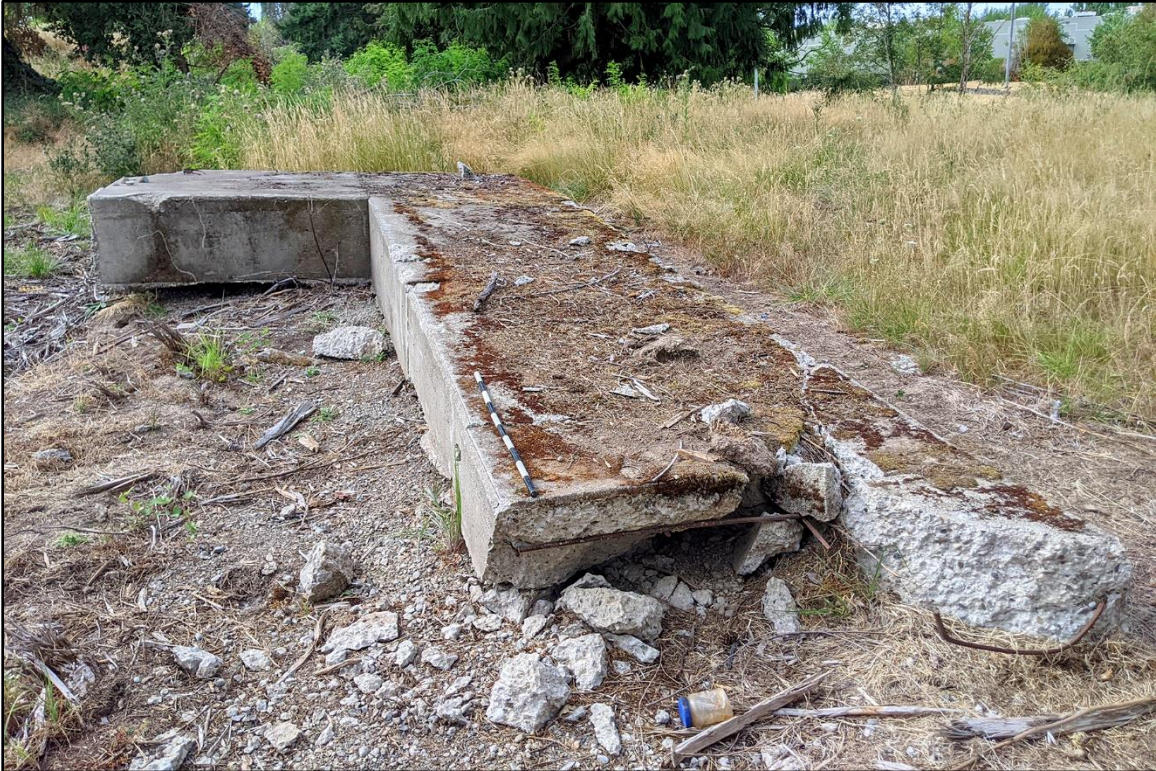
Figure 21. Remaining concrete patio from 1950s house. View to the northwest.
