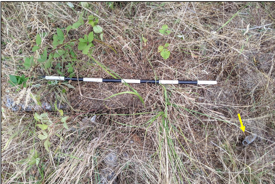
Figure 25. Close-up of 1950s outbuilding foundation (paralleling scale pole) and metal conduit pipe (marked by arrow).
