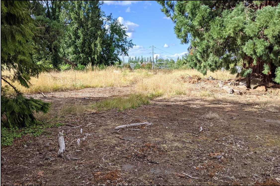
Figure 24. Overview of asphalt drive and parking pad at north end (edges marked by bushy grass). View to the northwest.
