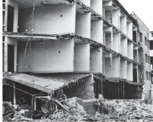
■ Figure 14. Heavily damaged Hotel Californian, 1925 Santa Barbara, California earthquake. —NISEE, U.C. Berkeley
