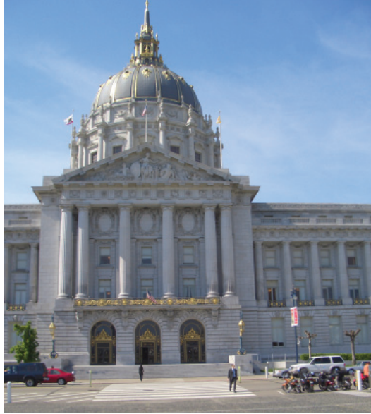
■ Figure 33. The San Francisco City Hall seismic retrofit, which includes seismic isolators. — Robert Reitherman
