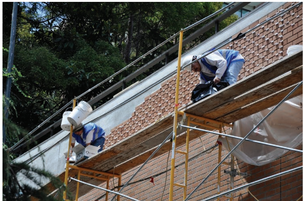
■ Figure 12. Workers installing brick veneer.
