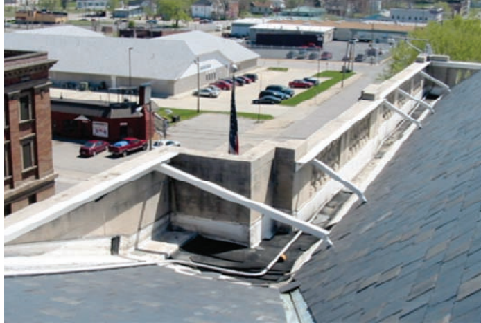
■ Figure 29. Retrofit bracing of an unreinforced masonry parapet.
