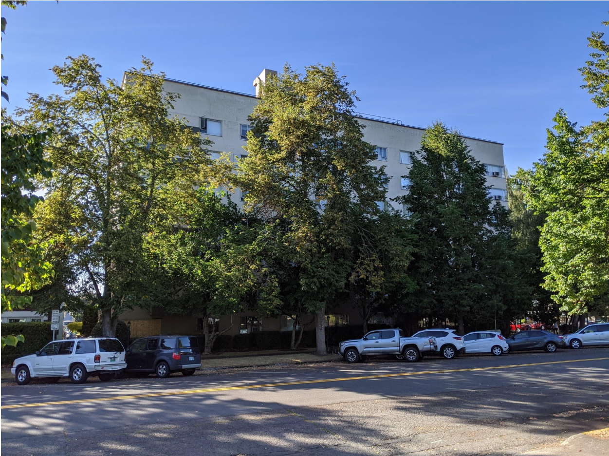
Front of the Lee Apartments from Winter Street NE. This building has several mature trees to protect it from the morning sun.
