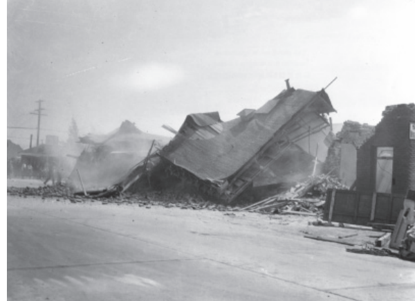
■ Figure 3. Complete collapse of an unreinforced brick building.
