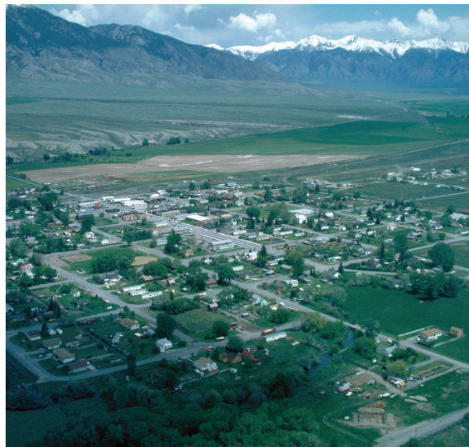
■ Figure 17. Aerial view of heavily damaged Mackay, Idaho. The unreinforced masonry buildings on the main commercial street of the small town were badly damaged in the 1983 Borah Peak, Idaho earthquake. —NISEE, U.C. Berkeley
