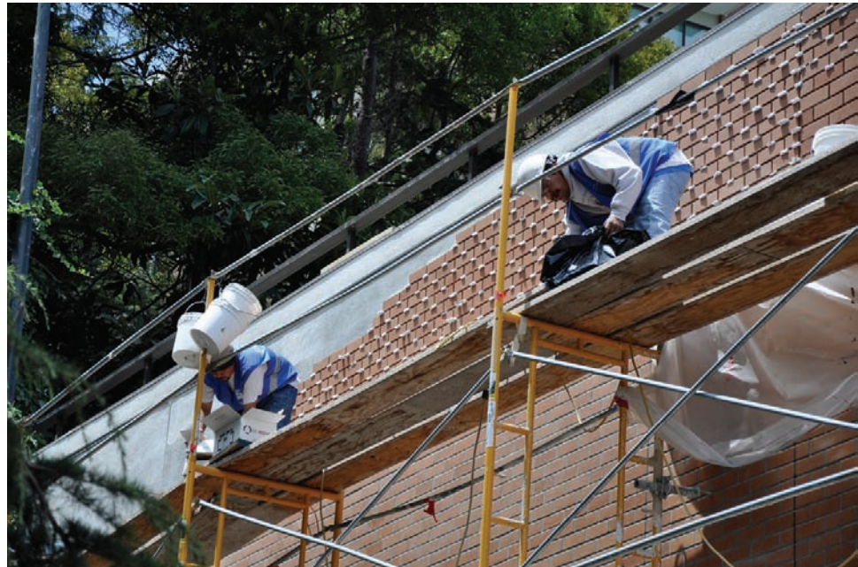
■ Figure 12. Workers installing brick veneer.
