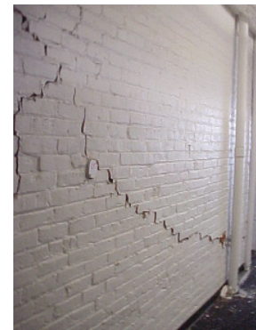
■ Figure 19. URM building damage, 2001 Nisqually, Washington earthquake.
