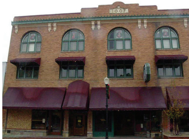
■ Figure 20. Retrofitted URM building, 2003 San Simeon, California earthquake.
