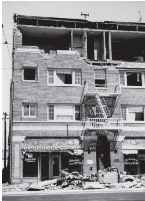
■ Figure 15. URM building damage, 1933 Long Beach, California earthquake. —Los Angeles County Public Library
