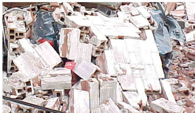
■ Figure 19. URM building damage, 2001 Nisqually, Washington earthquake.
