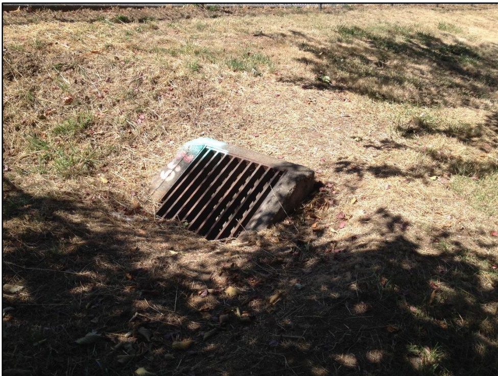
Photo Point 8: Catch basin next to Pringle Road SE
