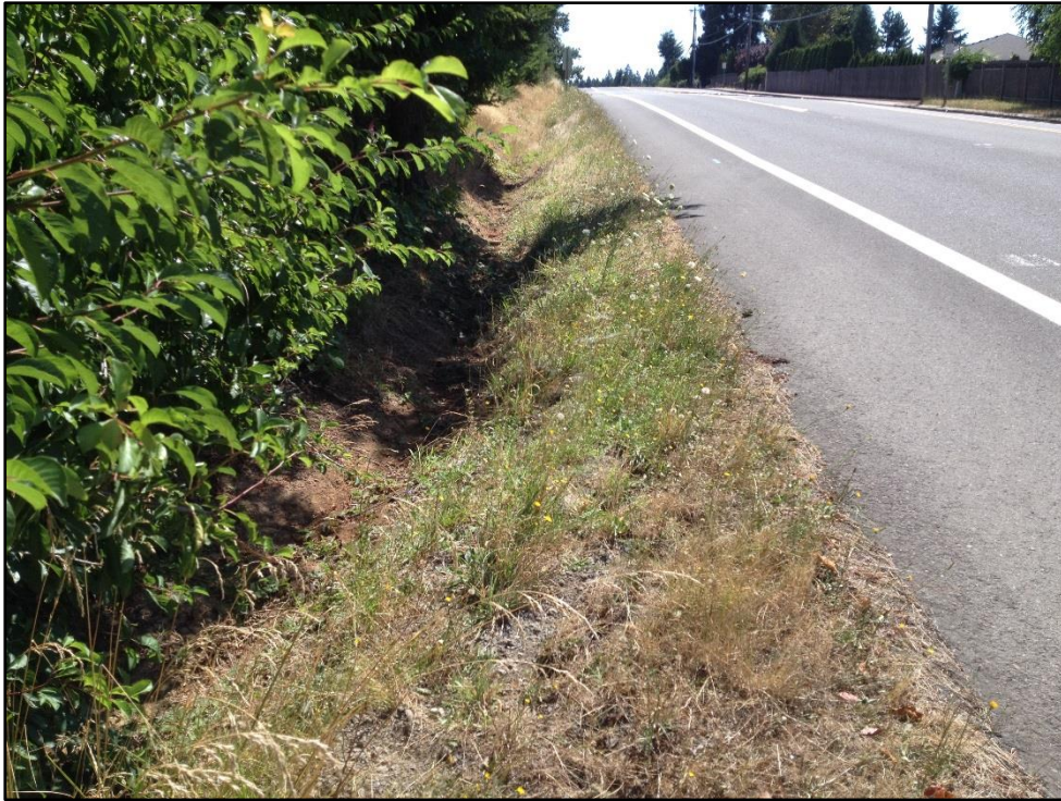
Photo Point 9: Roadside swale that intercepts runoff from Pringle Road SE
