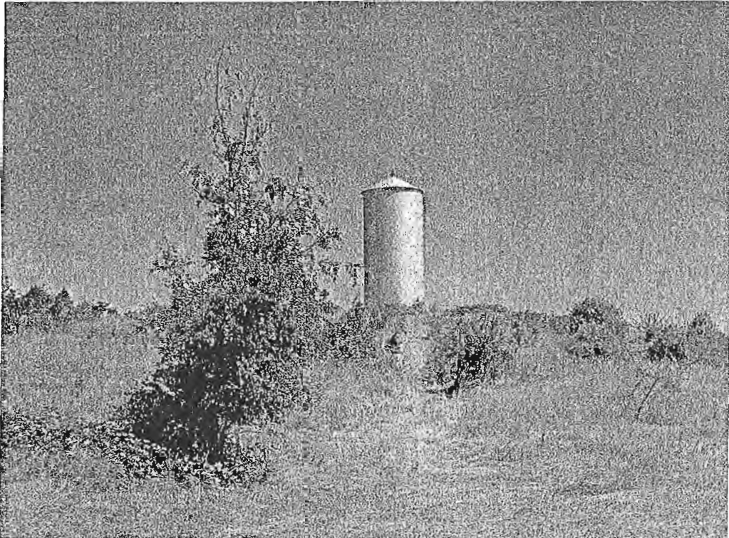
Figure 10: Looking northeast to water tower from orchard high grass area.
