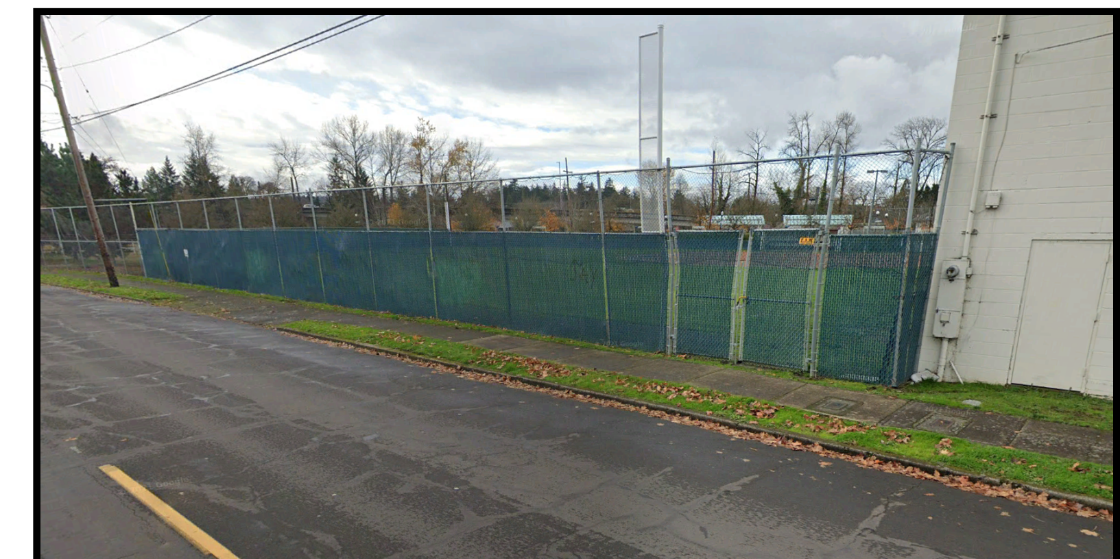
EXISTING FENCE AT BUILDING CORNER
