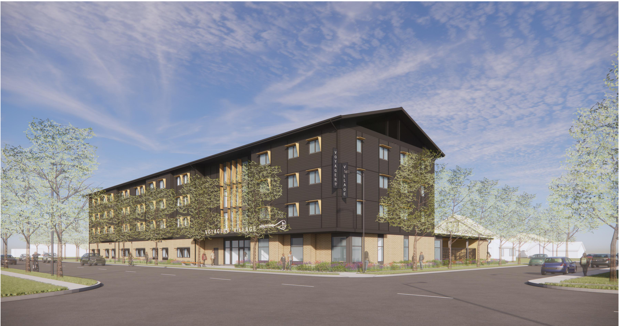
VIEW FROM SW
